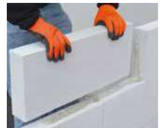
GASBETON® block laying
