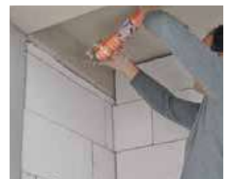
Thin vertical/horizontal joint sealing
