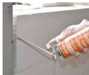
Thin vertical/horizontal joint sealing
