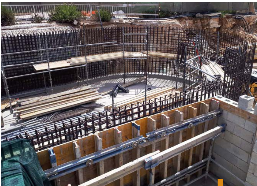
Creating the complex shapes of the pools in the Mediterraneo Marine Park required considerable skill in working with wooden formworks.
