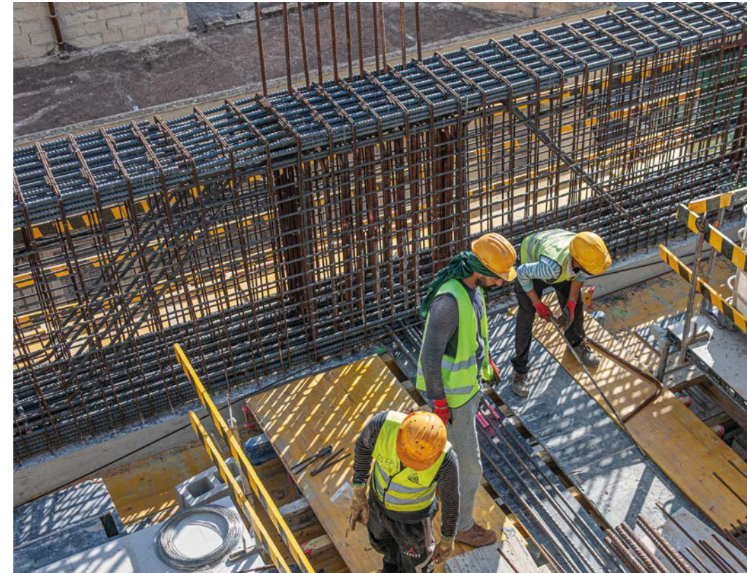
Massive steel reinforcement in a structural node at Regina Hotel construction site in Sliema managed by Attard Bros Group
